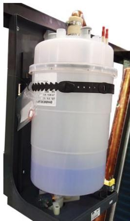
Modulating steam humidifier with immersed electrodes fitted with safety and running accessories. The optional is not available for size E1, E2.
