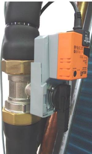
The water flow control in the finned coil is achieved through a **2-way modulating ball valve with equal percentage flow control** ensured by the integrated characterizing disc.
