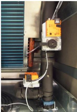
2-way motorized valve with 0÷10 VDC control actuator and emergency manual control for the third way (by-pass) of the hydraulic circuit.
