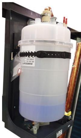
Modulating steam humidifier with immersed electrodes fitted with safety and running accessories. The optional includes the combined temperature / humidity sensor on unit air intake. The optional is not available for size E1, E2. The optional includes the combined temperature / humidity sensor on unit air intake. The accessory is factory installed and requires only water filling connection.
